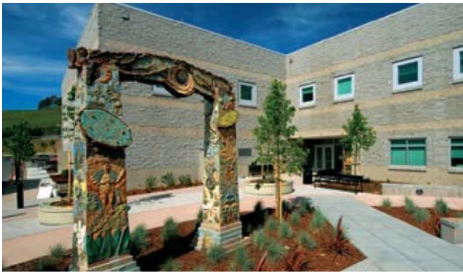
An 880-kilowatt rooftop solar system supplies 60 percent of the power needed to operate the Alameda County facility.
