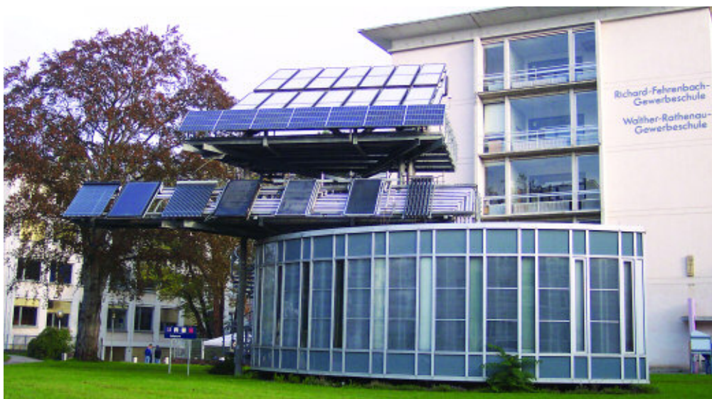
▲ THE EUREGIO SOLAR EDUCATION CENTRE serves as a practical tool for training electricians in the installation of solar-energy systems. It has many renewable energy systems on display outside of the classroom, thus providing information to the general public.
